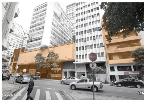
Figure 7 - Area 19. From the left to the right. First, Sol Belo Horizonte Hotel is a vacant building for commercial and/or services use. The hotel tower is vacant, and only the parking lot area is currently in use (Rennó, 2019). Second, Bahia Shopping (main entry) is a vacant building for commercial and/or services use. Only 500m 2 of its 10,000m 2 are being used for parking (Rennó, 2019). Third, there is a possibly underoccupied building for mixed-use. There are sale and rent signs on its facade. Source: Google Street View (Google Maps, 2024) [reference date: May 2019].
