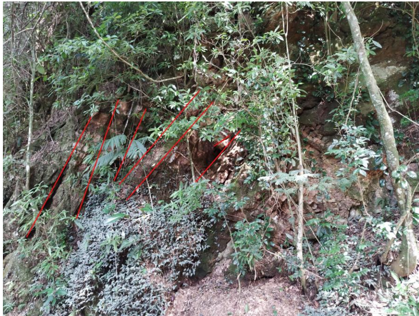
Figure 4 – Biotite-Gnaiss outcrop in an advanced stage of weathering with its high angle bedding leaning towards the road. Source: Authors (2022).
