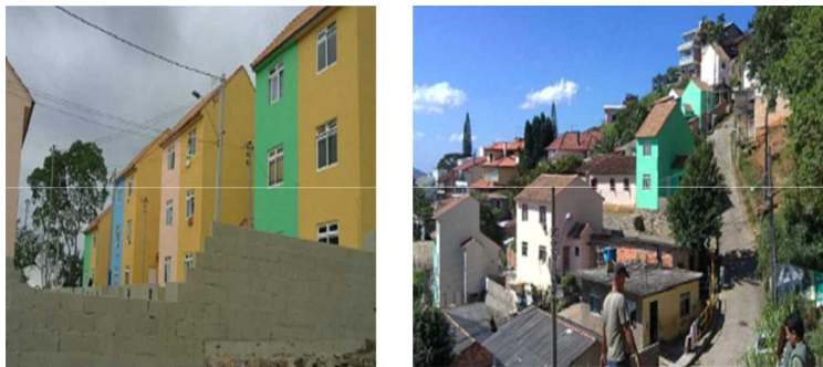
Figure 13 - Projects of Houses – Morro do Céu (location: arrow A on Figure 12). Source: Secretary of Housing and Environmental Sanitation-SMHA (Florianópolis, 2011).
