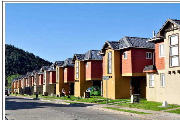
Figure 5 - Gated communities in the peri-urban area of Temuco
