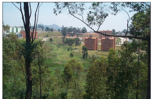
Figure 6 - Buildings of Sao Paulo State’s Urban Housing Development Company within the Pinheirinho d'Água Park Source: Charrette 2002 archive, in LABPARC digital archive (USP, 2002).
